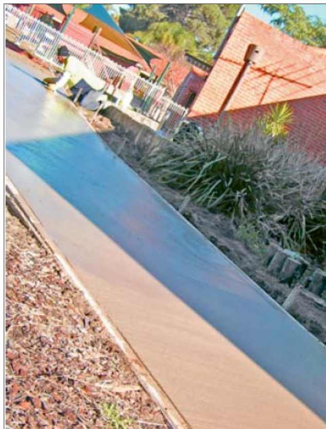
A geopolymer concrete path at Curtin University
