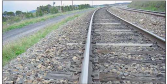
Figure 5 Geopolymer railway sleepers replacing some timber sleepers (photo courtesy of CSRP).
