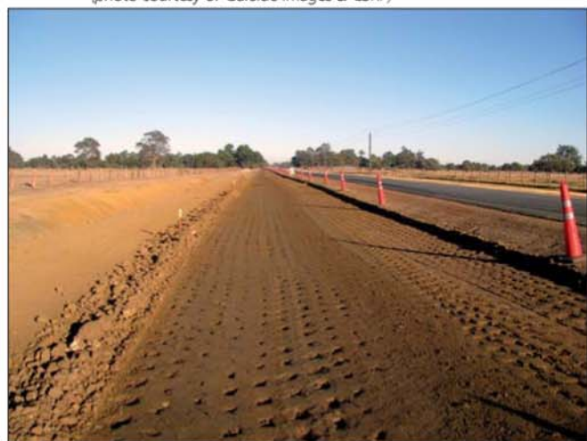
Figure 2 Road construction using ReSand ® as sub-base. (photo courtesy of DAFWA)
