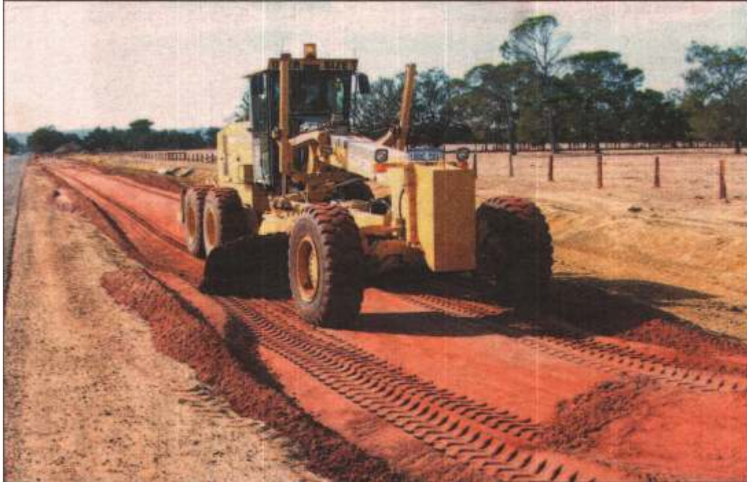
Alcoa's innovative new by-product is used in the construction of the new Perth to Bunbury Highway road network.
