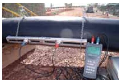
The ultrasonic meter used for site water meter calibration during the water audit at the Jundee mine © R. Cocks
