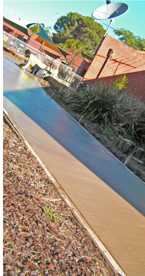
WA's first geopolymer concrete path at Curtin University (photo courtesy CSRP)
